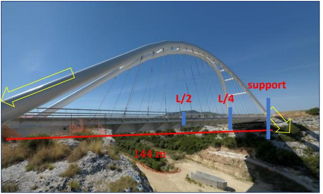
Bow – string bridge Steel-concrete deck 8 elastomeric isolators
