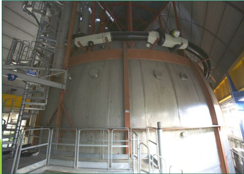
Before the thermal insulation (Mid 2015)
