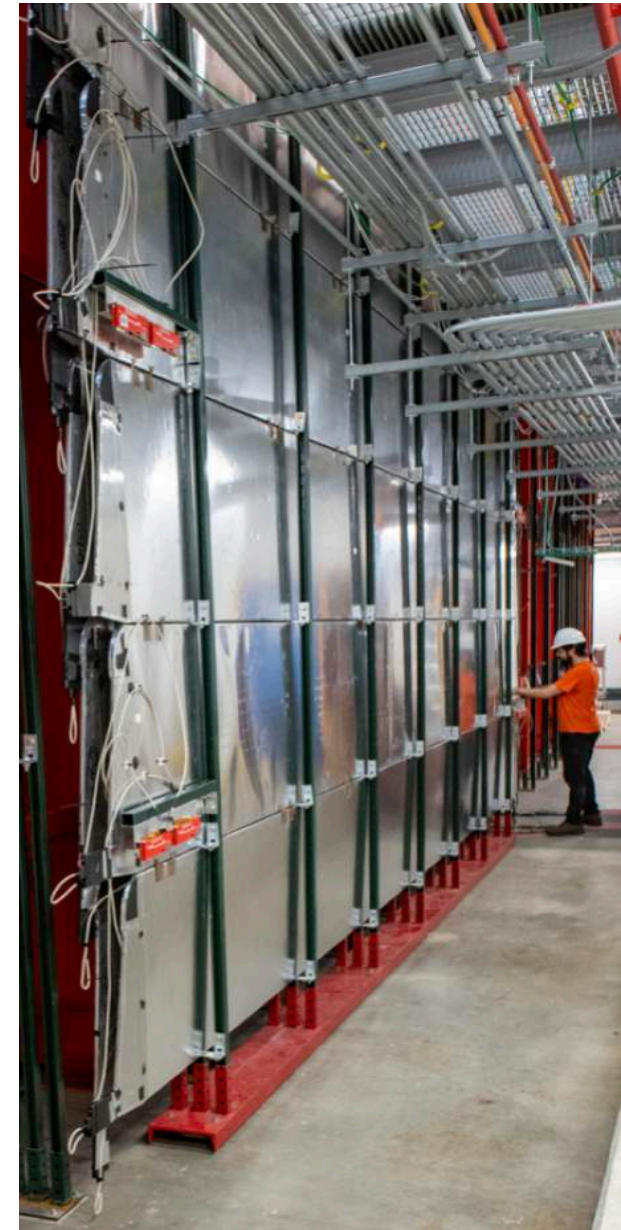
Side CRT partially installed
