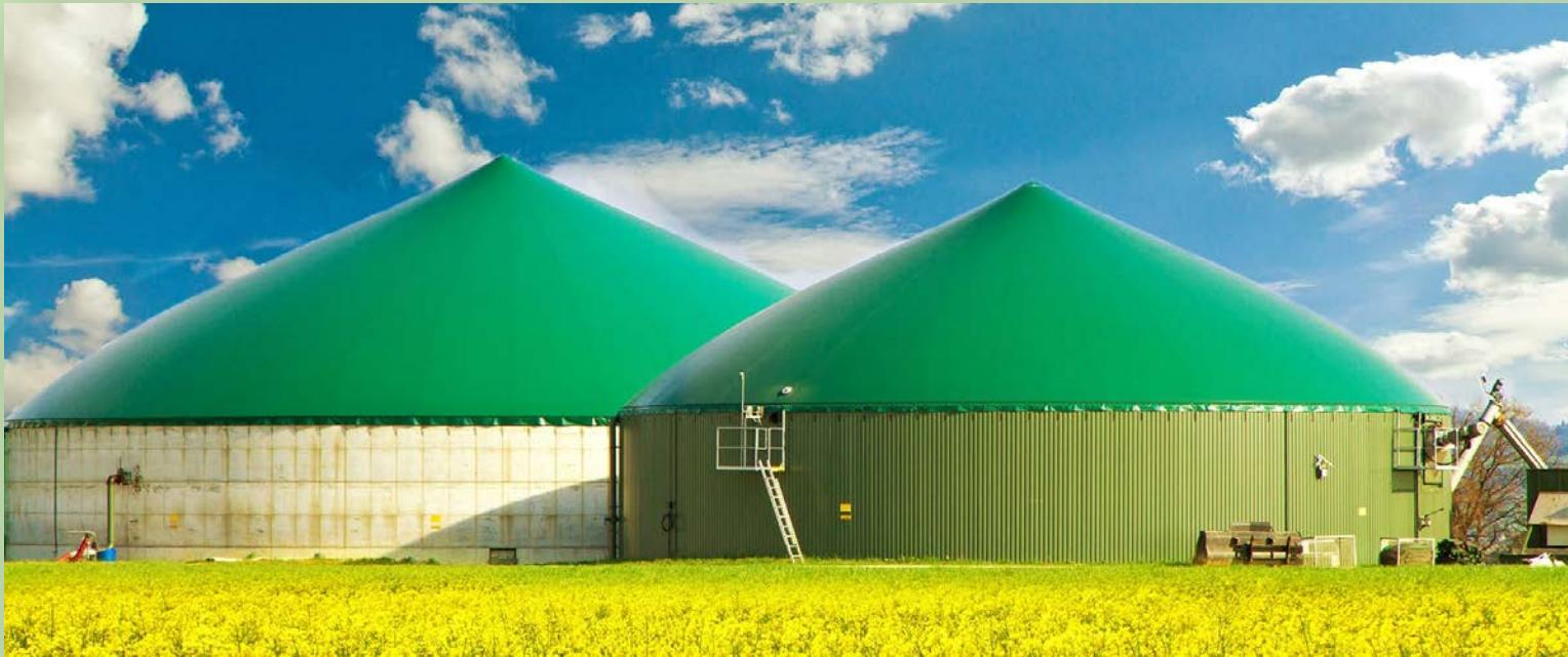
ANAEROBIC DIGESTION → Biogas → Mechanical energy → Electricity (Heat)
